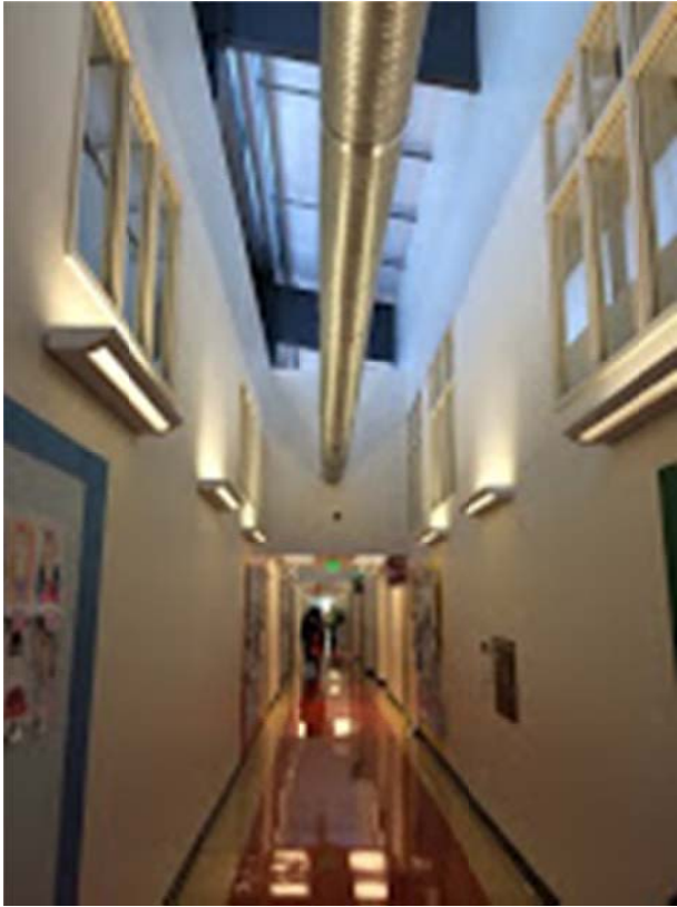
4. Second Floor Corridor
