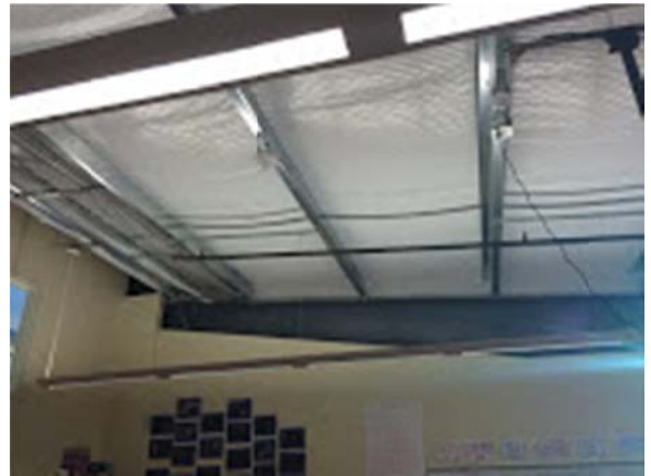
7. Second Floor Classroom Ceiling
