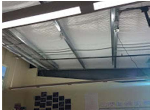
7. Second Floor Classroom Ceiling
