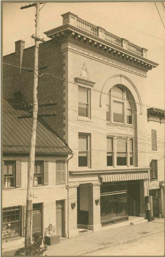
Historic Structure, Potomac Street Hagerstown, MD
